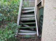
**Description:** Moderate wood decay damage was noted to timber structure at front of
